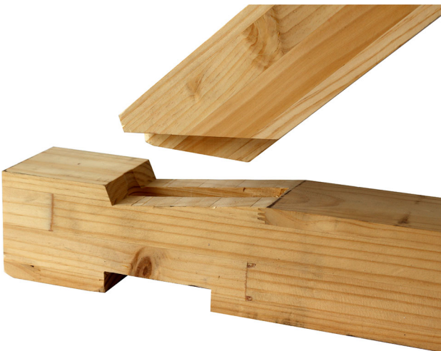
Fig. 8 Robotically milled oblique tenon joint
